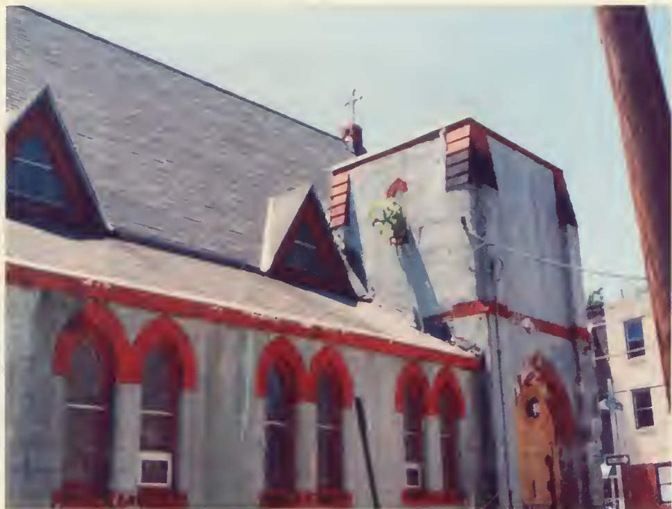
North Elevation of Church Building (H)
